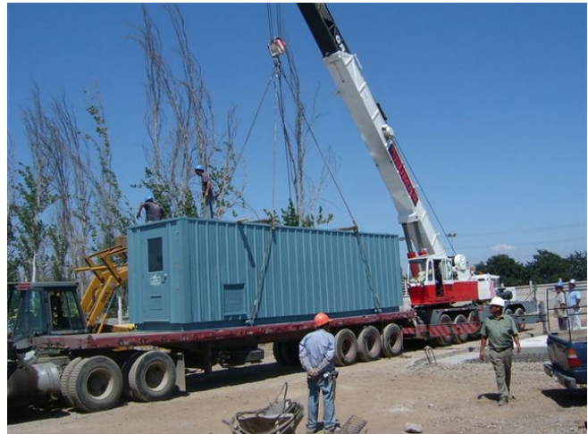
Photo 2: SNG Blending System being installed at Chile jobsite.
