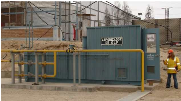
Photo 5: Typical Large Waterbath Vaporizer (Photo courtesy of Aprogas, Peru)
